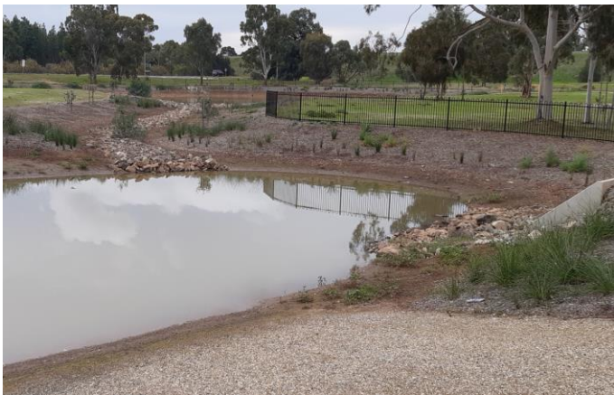
Jack Cooper Rise storm water Pond / Silt Trap/ buffer
