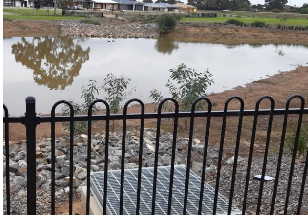
Jack Cooper Rise buffer pond with overflow grille
