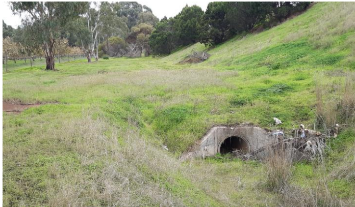
Swale running into s/w pipe to river
