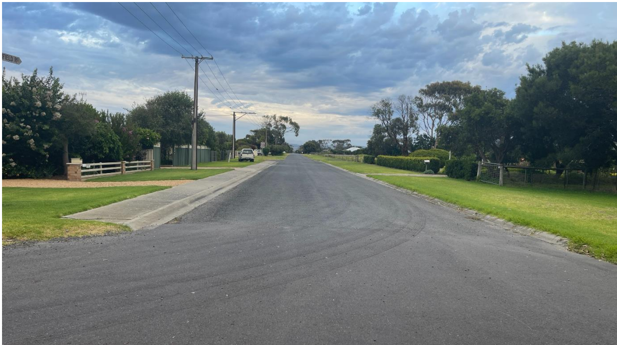
Figure 3.1: View West on Banfield Road (Affected Area on right)
