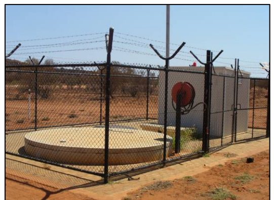
Effluent pump station
