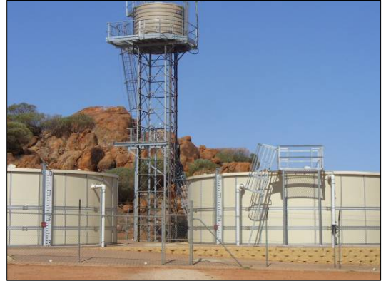
Water tanks and treatment facility
