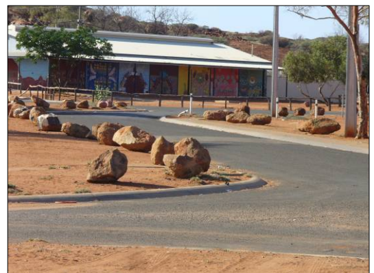
Sealed kerbed roads and rocks to control traffic
