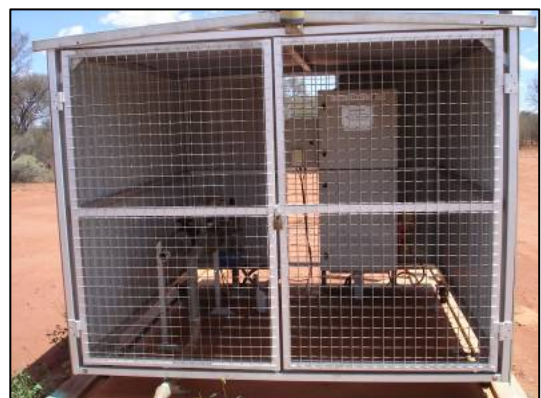
Water bore M1
