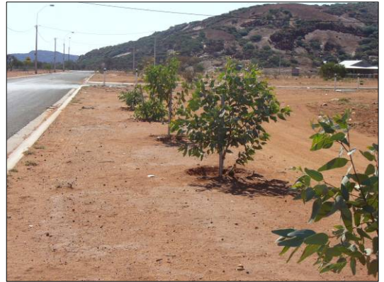
Road sealing and landscaping works are assisting with the reduction of dust
