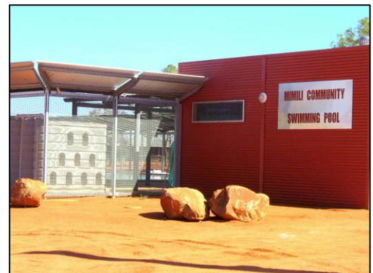
Rain water tanks at the swimming pool
