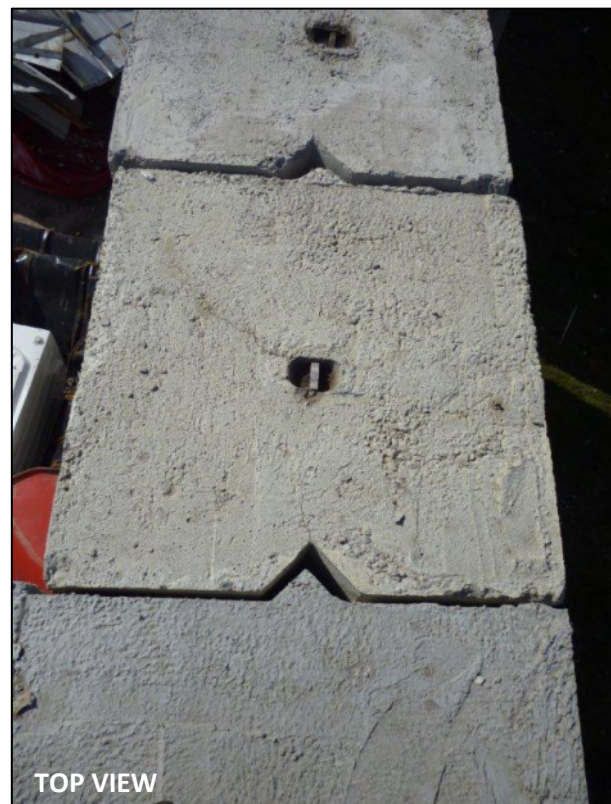
Photo 1.4b: Recycled Concrete block joins
