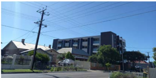
Figure 10: 'Tribeca building' Rankine Road. Urban Corridor. The imposing nature of this building has led to several residents selling their homes – homes in which they had invested a good deal of money. No tree canopy. Nevertheless, this building comprises about 10 fewer apartments than Ebor Avenue and two less levels.
