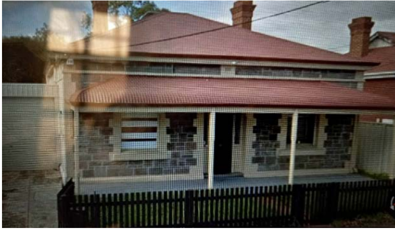
Figure 13 – demolished and not replaced.
