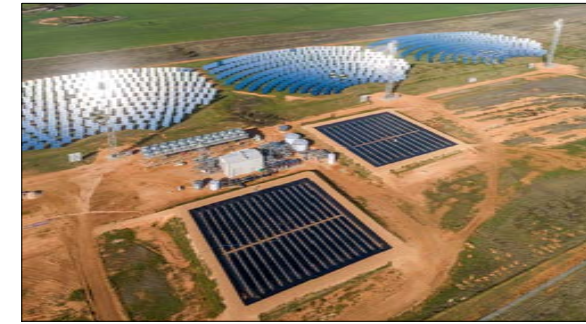
AERIAL VIEW OF SINGLE BLOCK DEVELOPMENT
