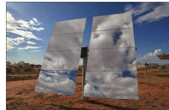
TYPICAL HELIOSTAT 5m x 4m
