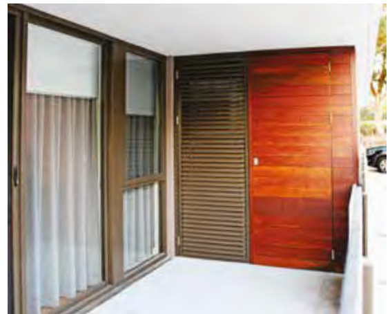
Photo 4.6b This storage area is integrated into the balcony design, weatherproof and screened from view.
