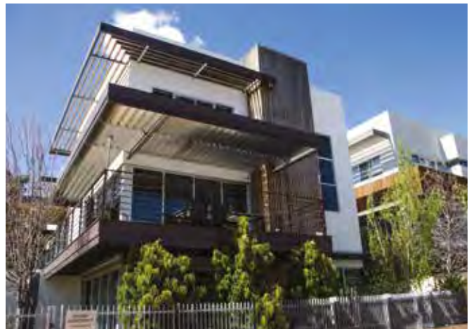
Photo 4.1f Different types of shading elements can adapt to the needs of different internal spaces and orientations. (PC)
