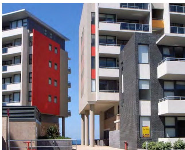
Figure 3F.7 Solid walls with non-habitable room windows are used for end elevations to manage privacy impacts between buildings. Solid balconies at lower levels provide better privacy from the street
