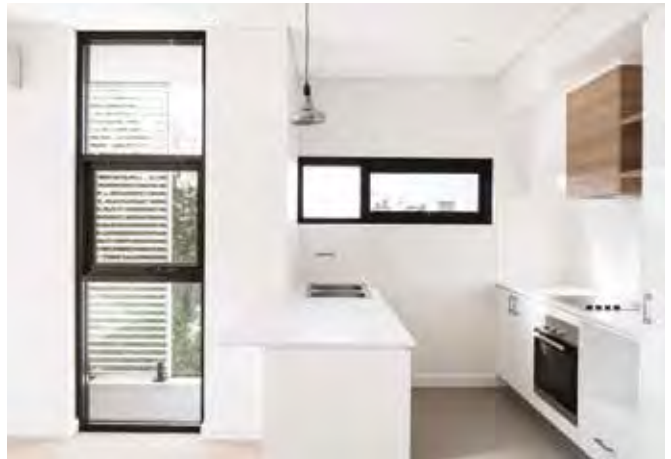
Photo 4.2b, c & d (From top) Louvre, casement and awning windows are preferred to sliding windows as the latter provide limited opportunity for the control of breeze. (PC)
