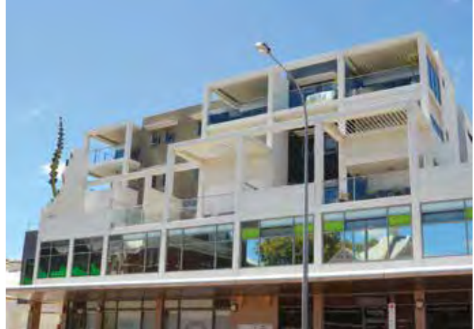
Photo 4.1d Shading and glare-control measures help to moderate solar gain for west-facing windows and balconies, including operable roof louvres to optimise sunlight and shelter.
