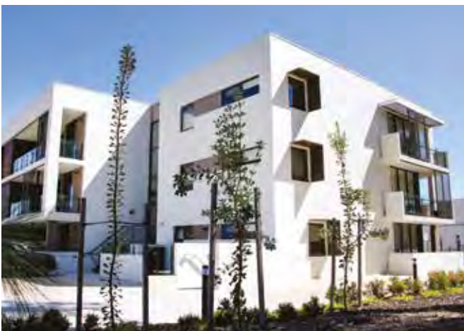
Photo 4.1e Simple sun shading device can be effective in minimising heat and glare. (PC)
