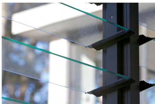
Figure 4B.7 Operable louvres allow residents to regulate natural ventilation
