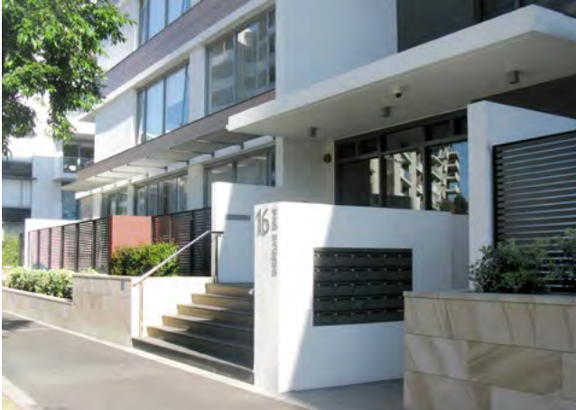
Figure 3G.4 Features such as awnings, blade walls and signage contribute to building entries that are clearly identifiable from the street
