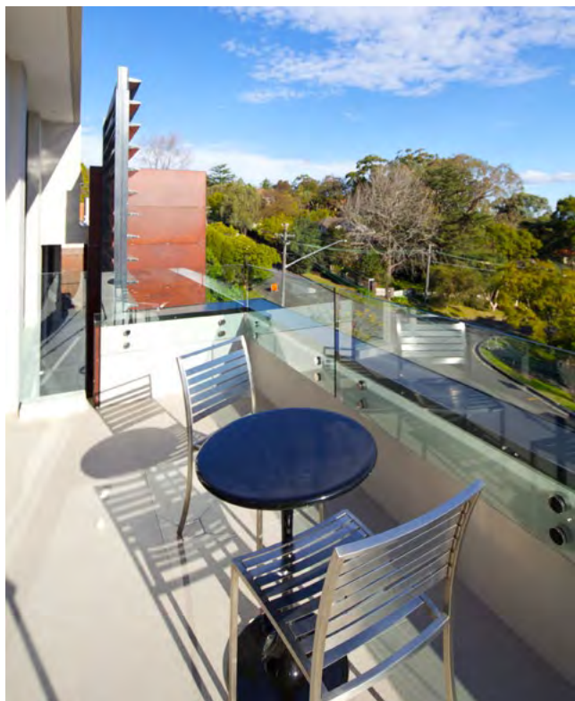
Figure 4E.6 For one and two bedroom apartments, balconies should be at least 2m deep to allow enough space for a small table
