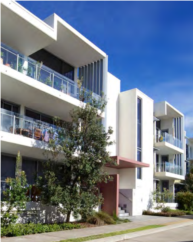
Figure 4C.4 Differing ceiling heights are an opportunity to provide visual interest in the building facade
