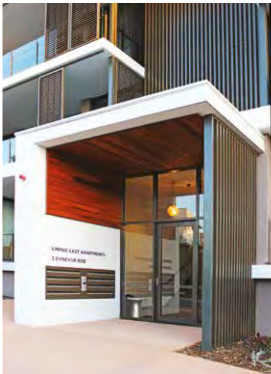
Photo 3.7a An entrance portico offers shelter, security and a recognisable point of address.
