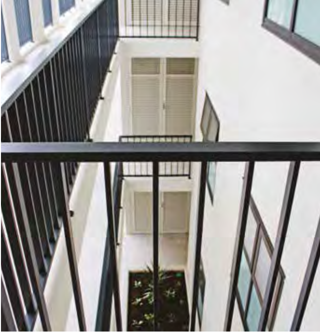
Photo 4.5d Communal walkway is separated by a void from dwelling windows to provide some degree of privacy.
