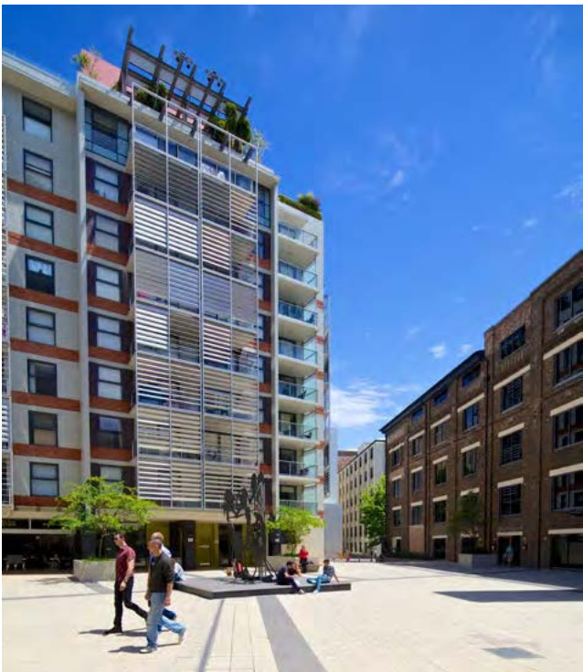
Figure 3D.13 This semi-public courtyard connects to the surrounding inner-city neighbourhood and offers a central water feature, seating and convenient pedestrian through-site links
