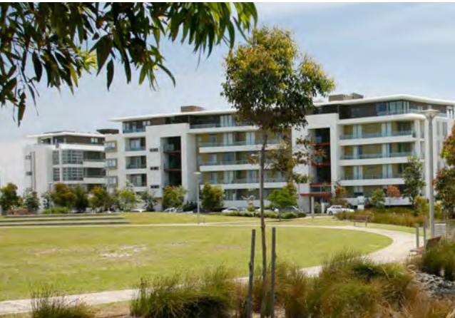
Figure 3D.9 Communal open space and public domain should be readily visible from habitable rooms and private open space areas while maintaining visual privacy
