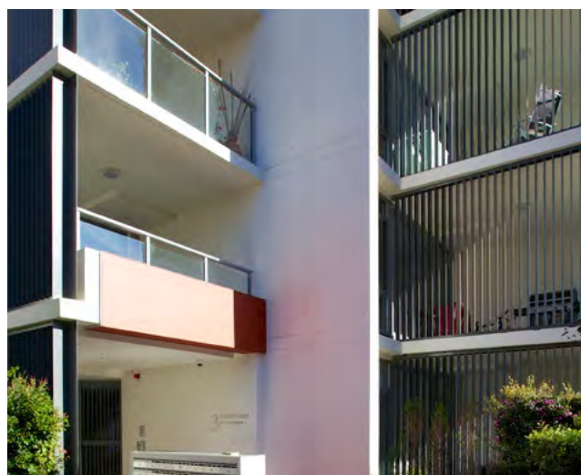
Figure 3F.8 Well designed fences and balconies provide privacy to apartments when viewed from the public domain or adjacent apartment buildings
