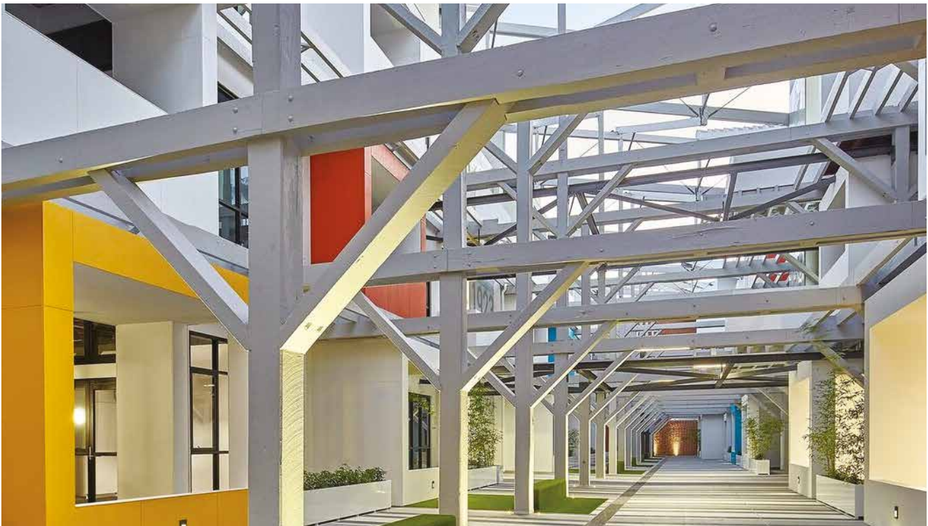
Photo 4.5f The roof and floors in the middle section of this adaptive reuse of a heritage building have been removed to allow for better natural ventilation and light to reach the circulation area. (PC)
