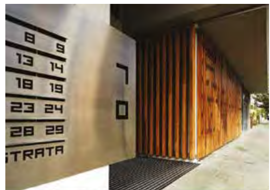
Photo 3.7c Signage should respond to the context and desired streetscape character. Here the building address signage has been integrated as a feature of the façade design. (PC)
