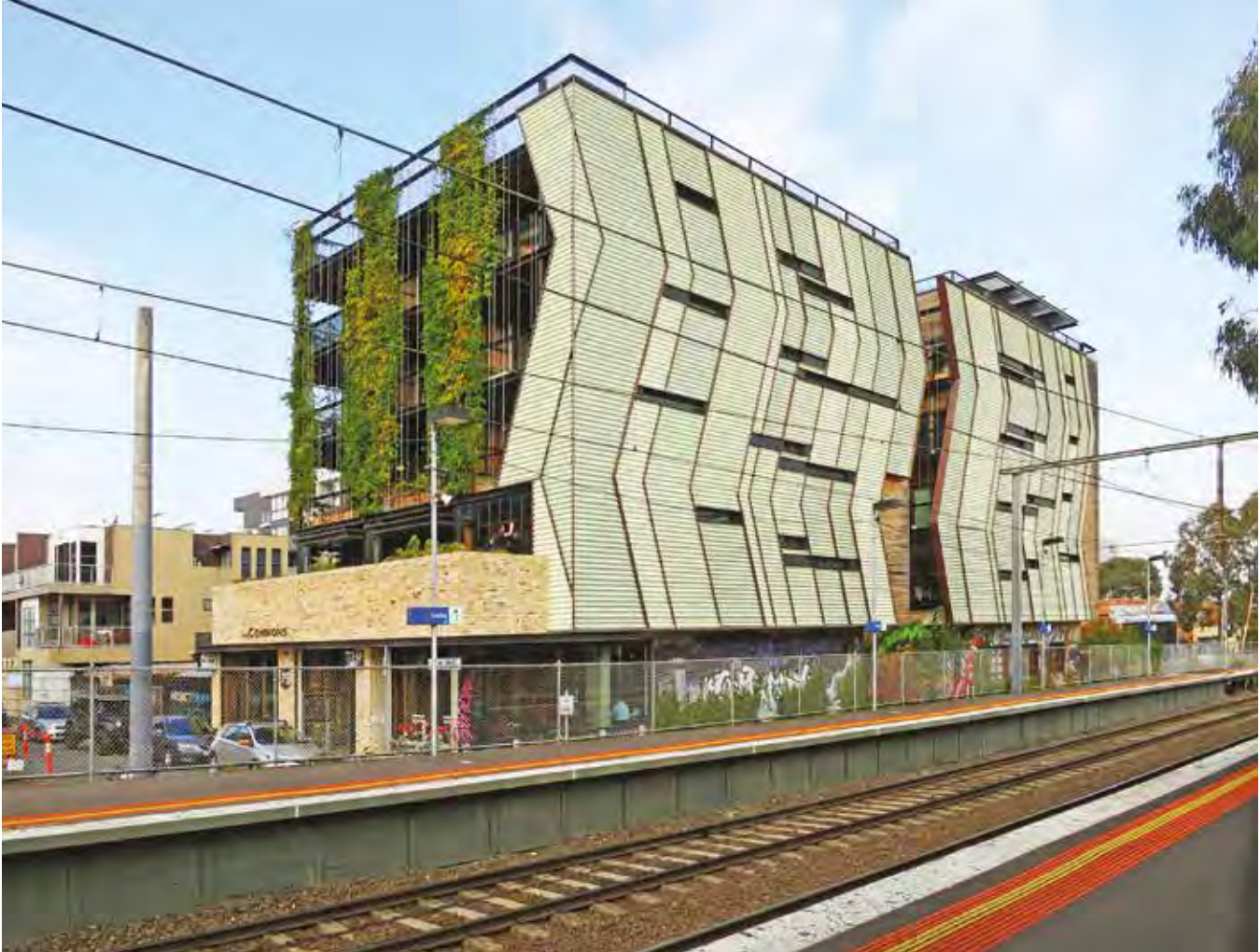
Photo 4.7a By considering noise sources in the orientation of the building and the design of façades and windows, good living conditions can be achieved even in close proximity to noise sources.
