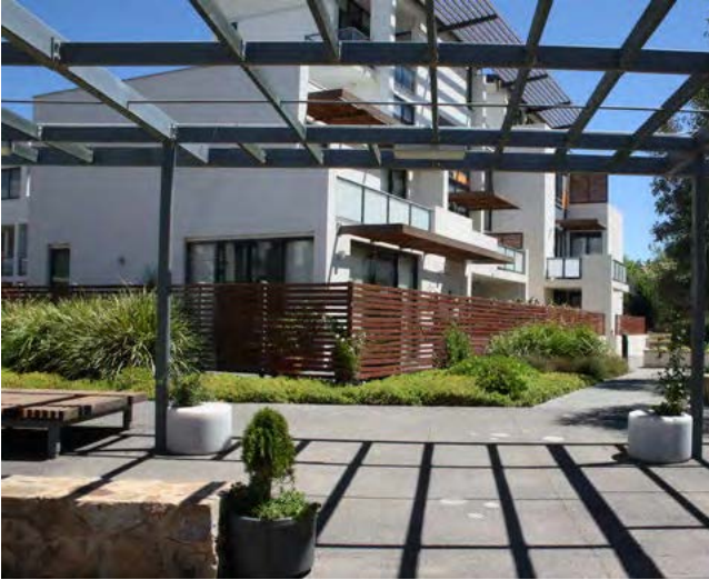
Figure 3D.12 This communal courtyard provides gathering spaces, seating facilities, pergolas and barbecue facilities for residents
