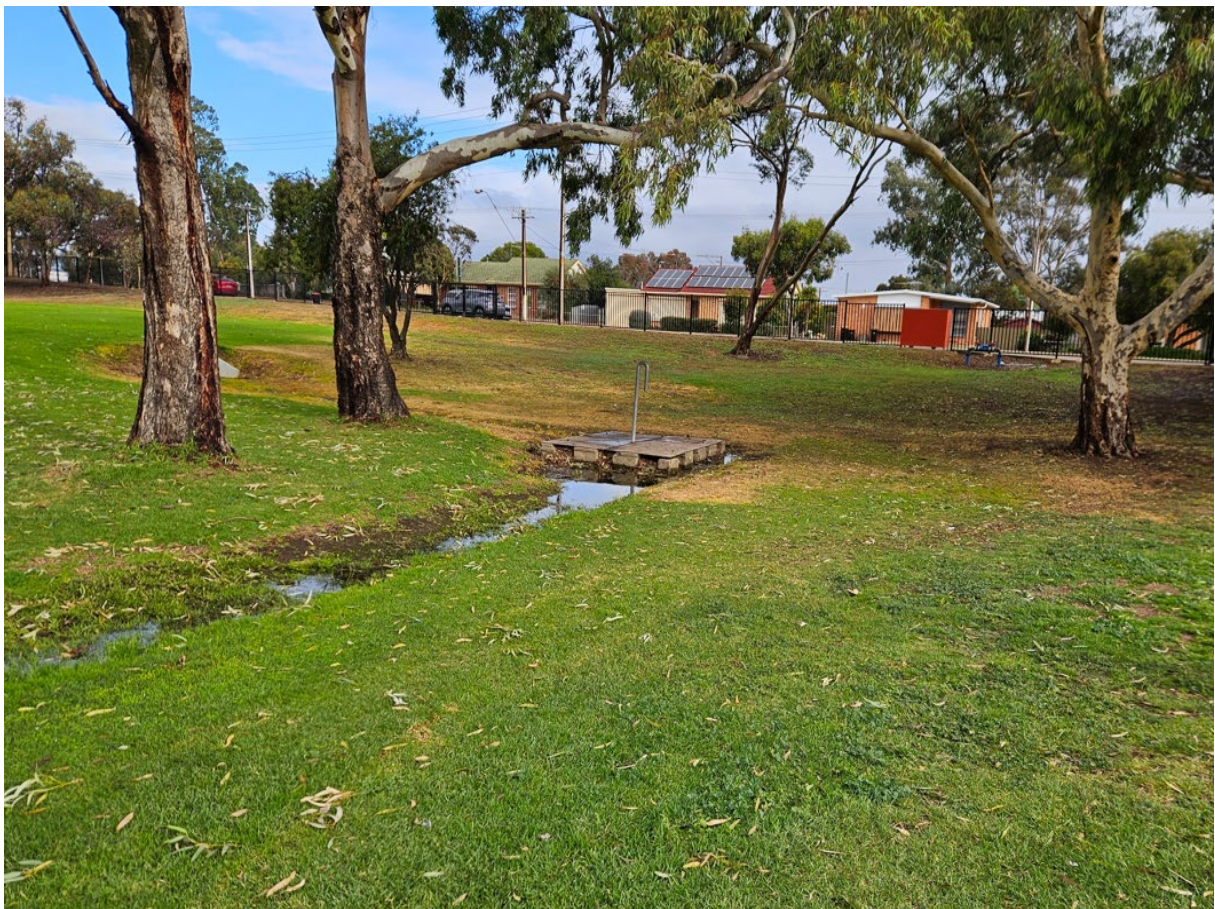
Photo 4: Showing the existing drainage basin and associated drainage bore.
