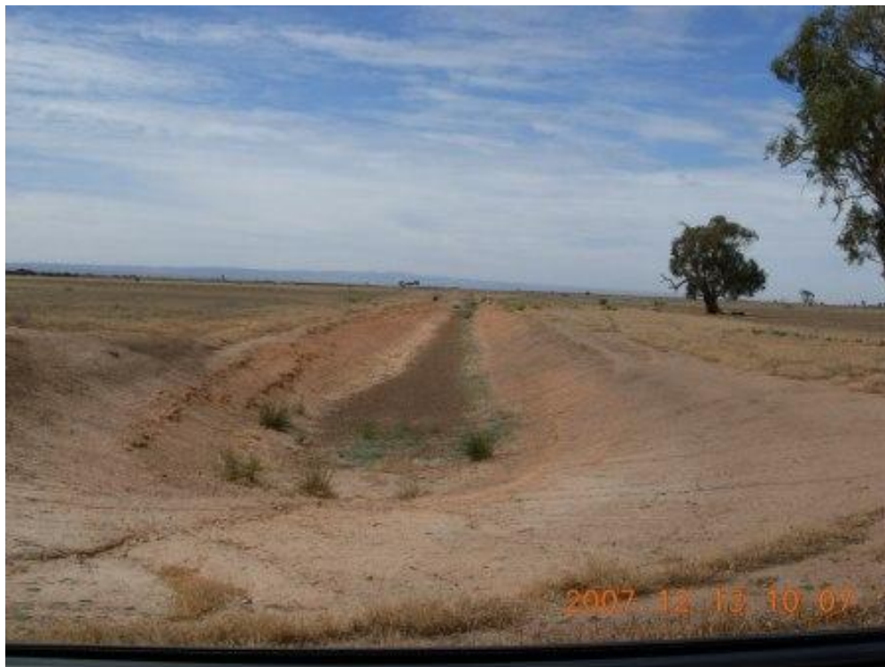
Figure 4-10: Failed irrigation system south of Gawler River, mid-way along the northern boundary of North Sector East
