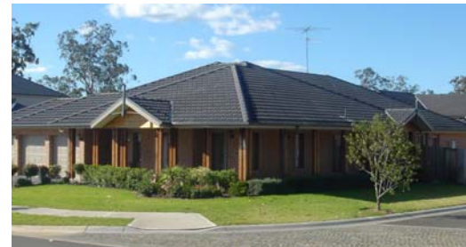
Corner house addressing both street frontages
