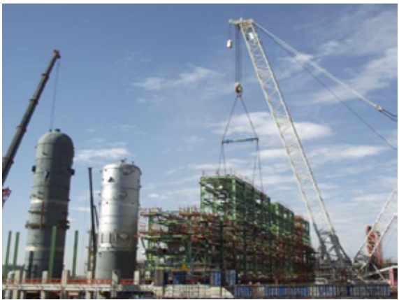
Pre-Assembled (PAR) Pipe rack and/or Conveyor Gallery
