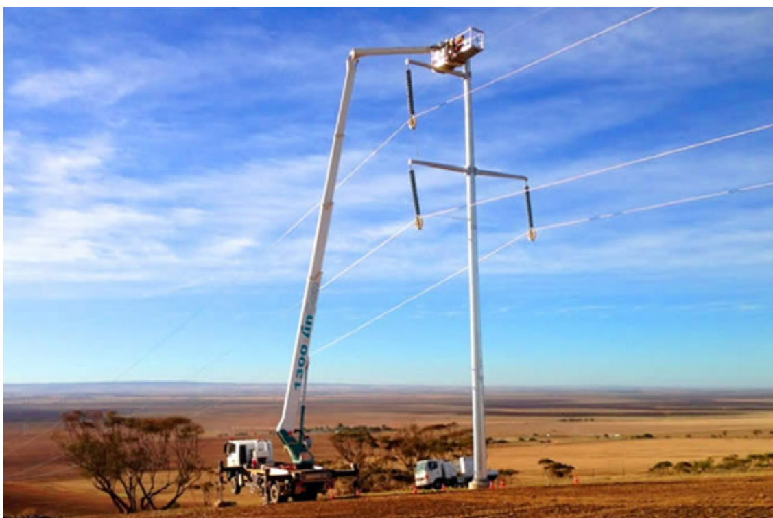
Figure 4-16 Example of Steel Monopole
