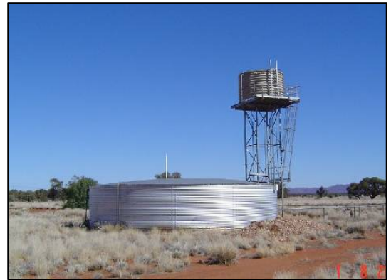
Water storage tanks and new electric bore
