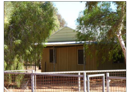
Typical community house
