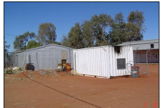
Nyapari power generation compound
