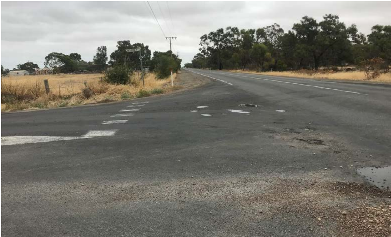
Gawler Road / Bethesda Road intersection (view west)
