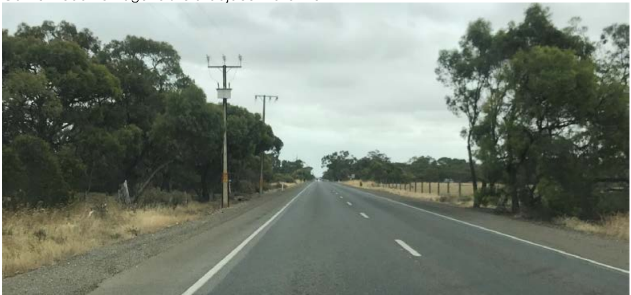
Gawler Road approach to Bethesda Rd intersection (view west)
