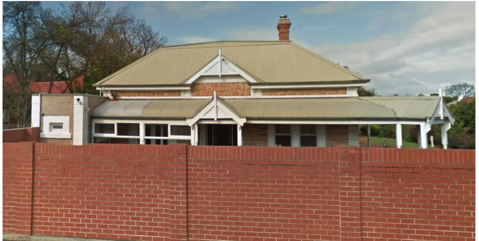
Figure 6: 5 Nottage Terrace, Medindie. Source: Google Street View, Aug 2016
