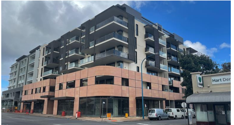
Figure 12: 244-248 Unley Road, Hyde Park, viewed from Unley Road
