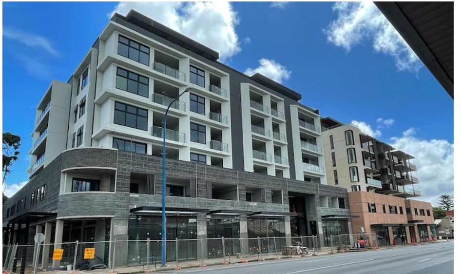
Figure 13: 244-248 Unley Road, Hyde Park, viewed from Unley Road
