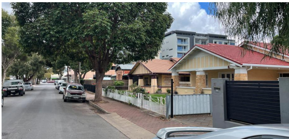
Figure 15: 244-248 Unley Road, Hyde Park, viewed from Hart Street within the Historic Area Overlay
