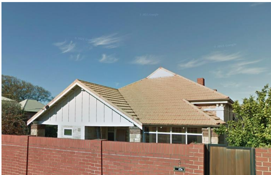
Figure 4: 3 Nottage Terrace, Medindie. Source: Google Street View, Aug 2016
