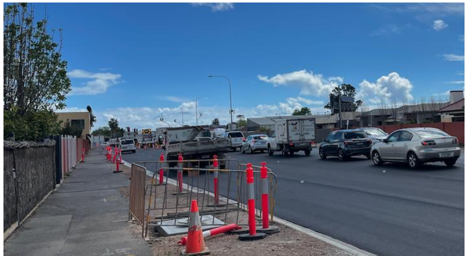
Figure 9: Nottage Terrace approaching Affected Land (left)
