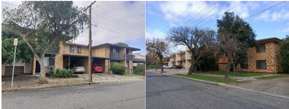
Figure 15 – Modern two-storey development located within eastern area of Glandore Character Area. Their impact to the area’s character is negligible due to them being few and far between.
