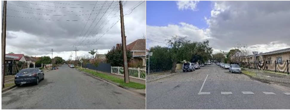
Figure 13 – Street views from Weymouth Avenue, image on right looking toward Anzac Highway. The photos display that the area currently has clear skyline/ rooflines and the street trees do not dominate the area or alter the roofline. This allows the area’s character to be displayed and help form its streetscape, which could be harshly impacted by eight-storey developments.
