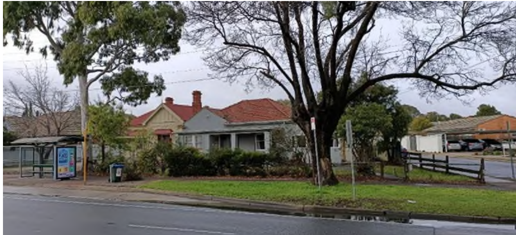
Figure 1 – 118A Anzac Highway
