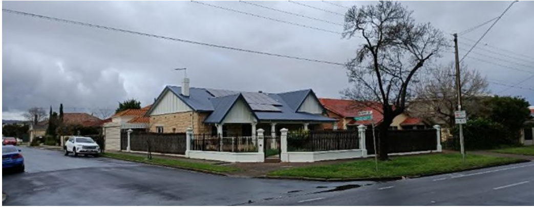
Figure 4 – 158 Anzac Highway (dwelling with blue roof)
