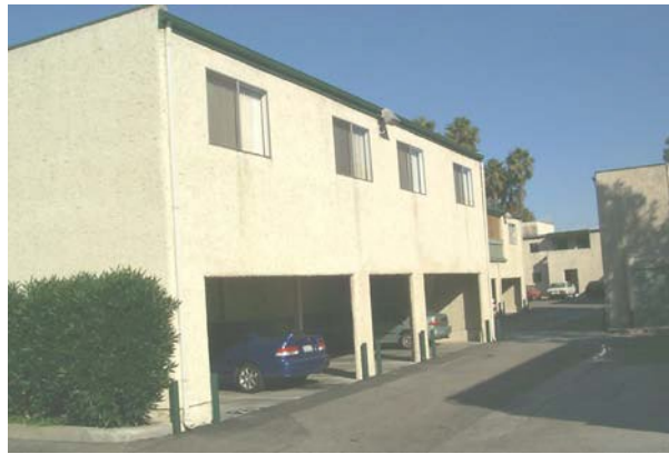
Figure A1-03 - Example of soft storey conditions, where parking requirements result in large weak openings.
