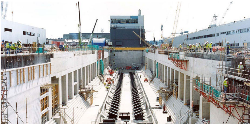
Figure 5.4 - 9 Dock at Devonport in the United Kingdom (Source: Navy Lookout 2020)
