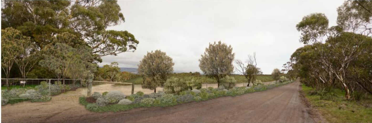
VIEW OF DAM PROJECT 5 YEARS AFTER CONSTRUCTION
