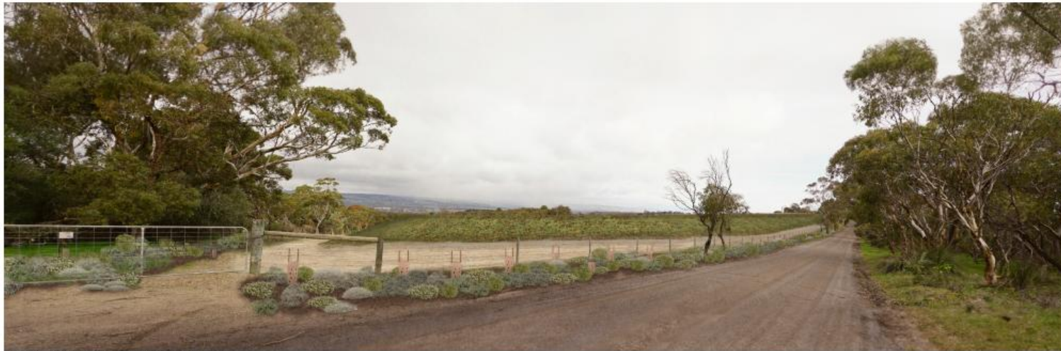
VIEW OF DAM PROJECT POST CONSTRUCTION (1 YEAR)
