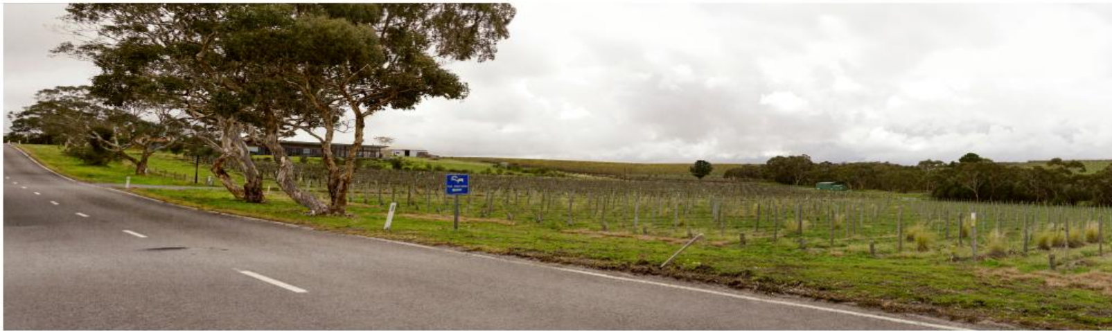
VIEW OF DAM PROJECT POST CONSTRUCTION (1 YEAR)
