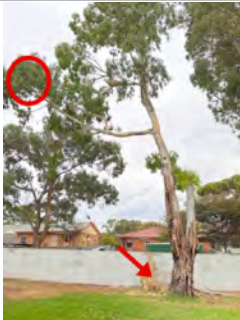
Photo shows failed limb to mulch and western lateral to reduce.
