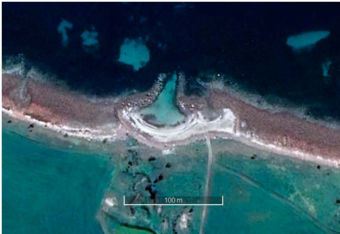
Figure 3-13 Rock groynes constructed by shifting local material
