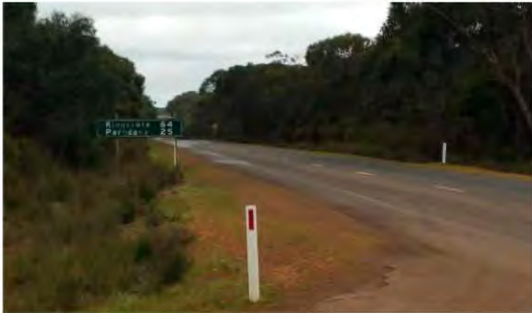
Figure 11. Sightlines Obscured by Sign
