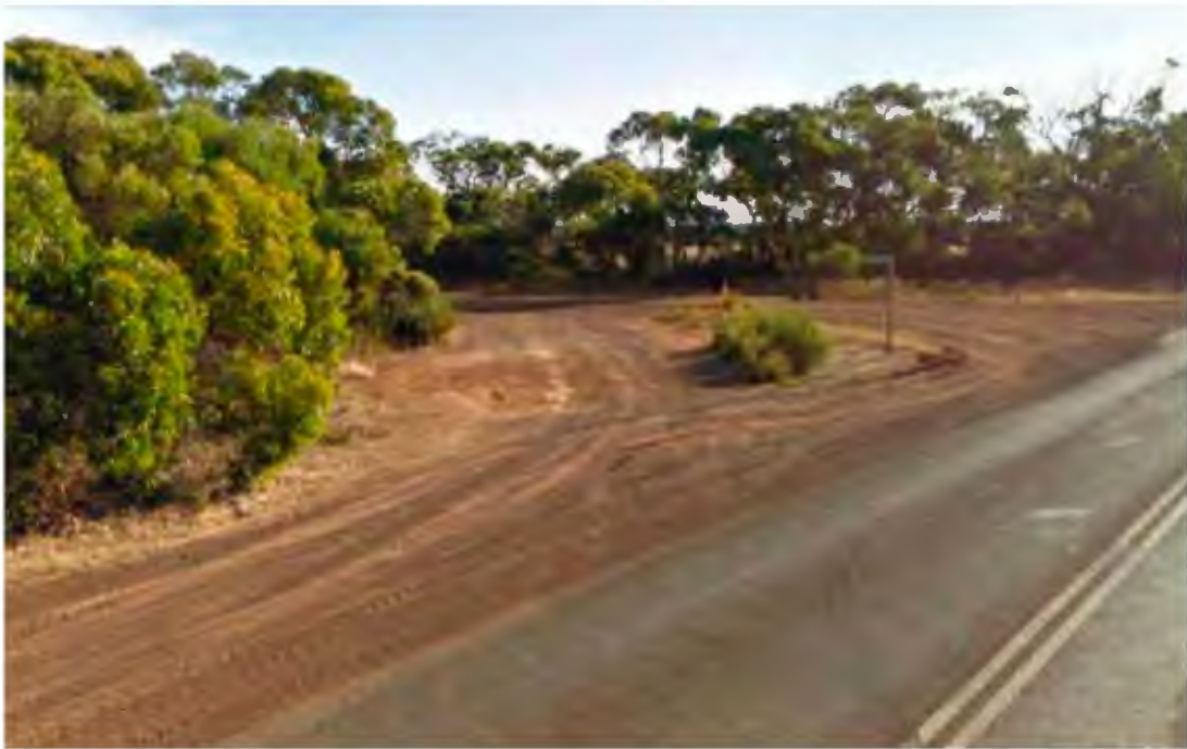
Figure 12. Informal Left Turn Arrangement, Playford Highway Western Approach
