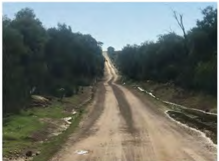
McBrides Road 2 - insufficient drainage
