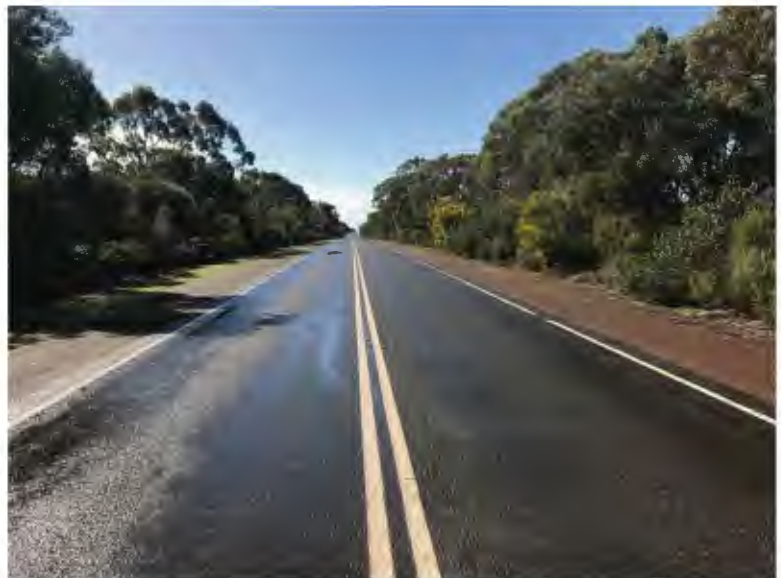
Playford Highway 4 - evidence of seal delaminating
