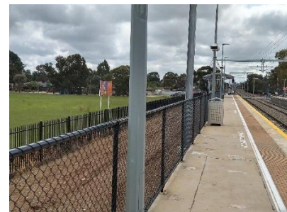
Photo 3: Western access to the station via the main road
