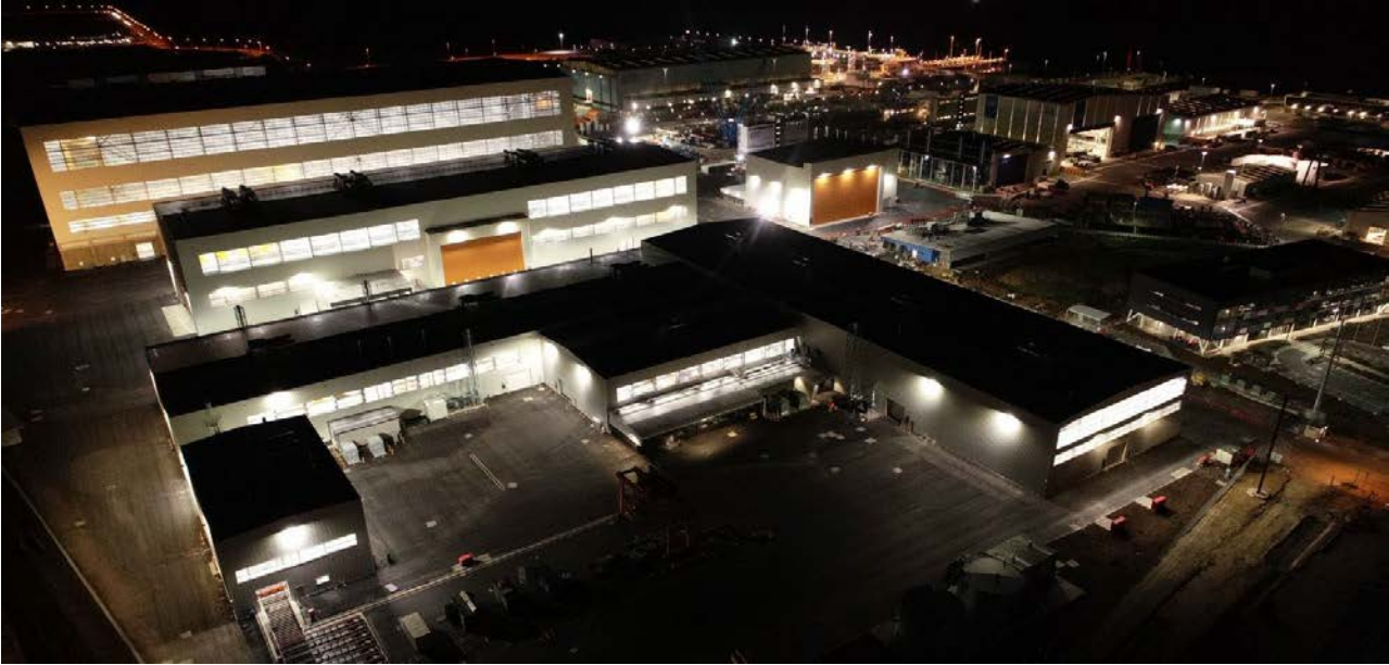
Figure 19: Lighting at existing Osborne Naval Shipyard (Source: Australian Naval Infrastructure 2020)
