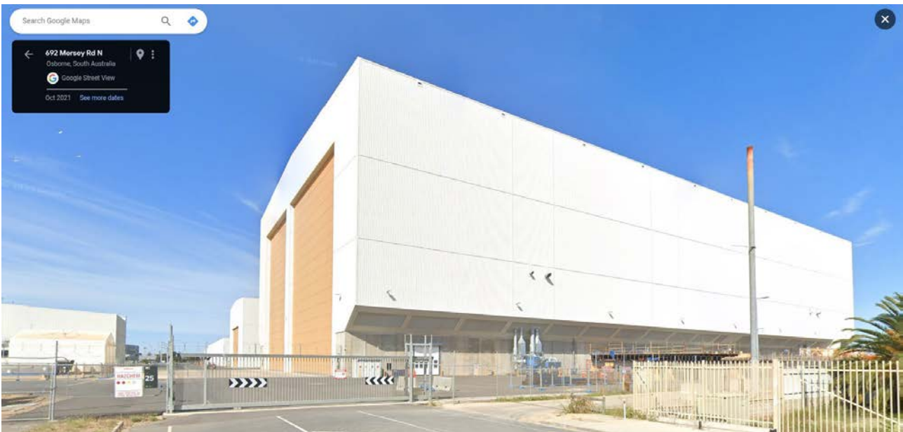
Figure 17: Close up view of a large fabrication hall at the existing Osborne Naval Shipyard.
