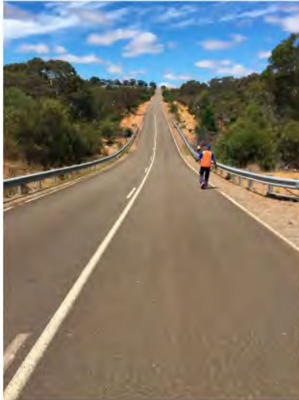
Photo No. 5 – Item 4, guardfence protecting the culvert, the dip is very tight.
