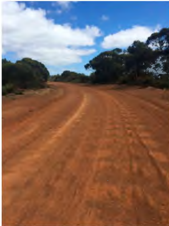
Photo No. 32 – Item 104, corrugations and tight horizontal curve.
