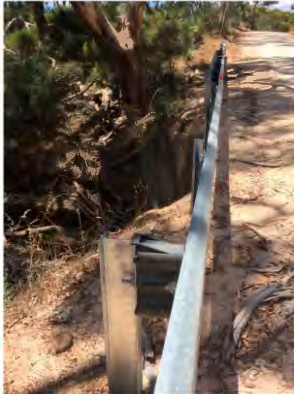
Photo No. 7 – Item 12, guardfence protecting a deep culvert close to the carriageway.
