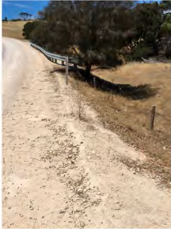
Photo No. 13 – Item 43, guardfence protecting a culvert, batter slope not covered.
