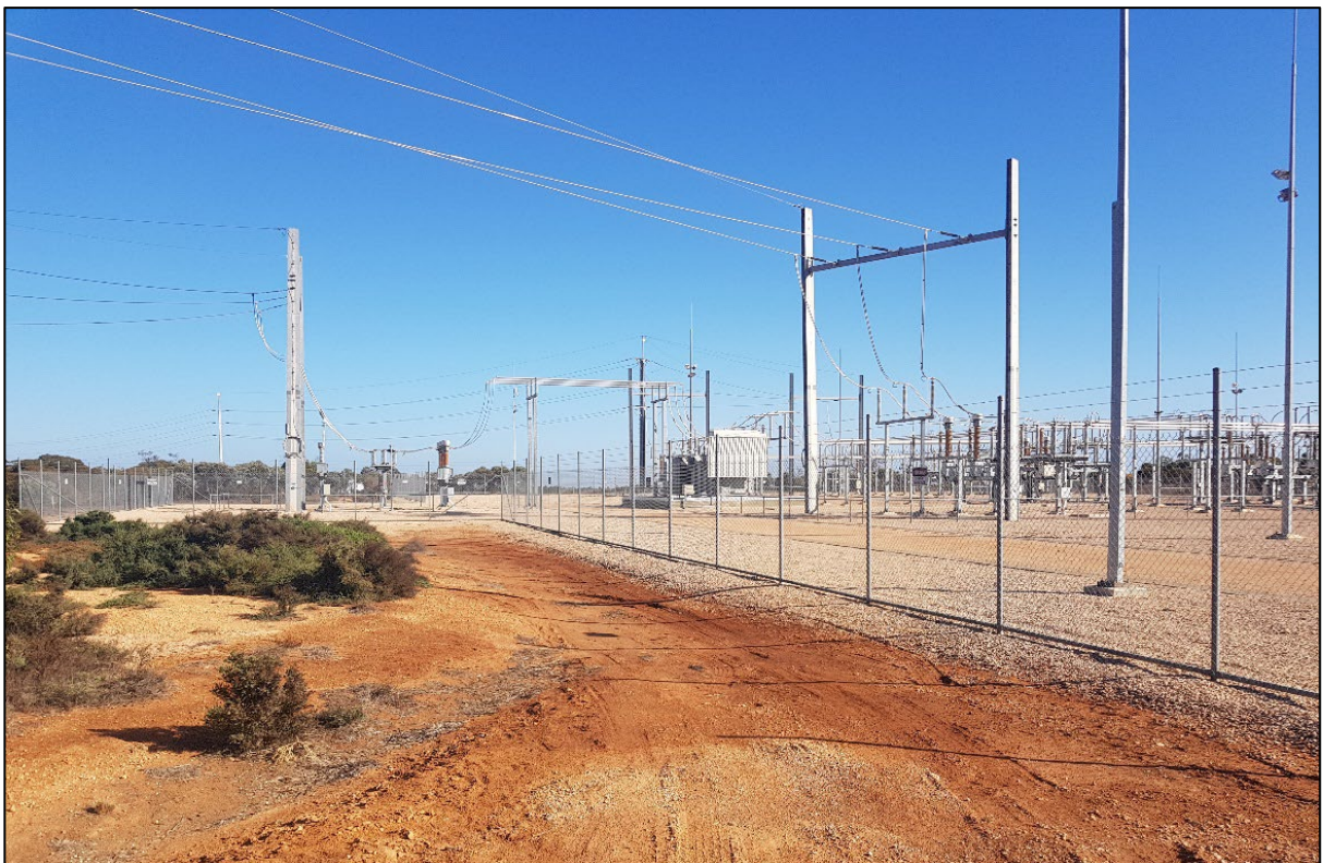
Figure 2: Monash Substation as viewed facing north-west
