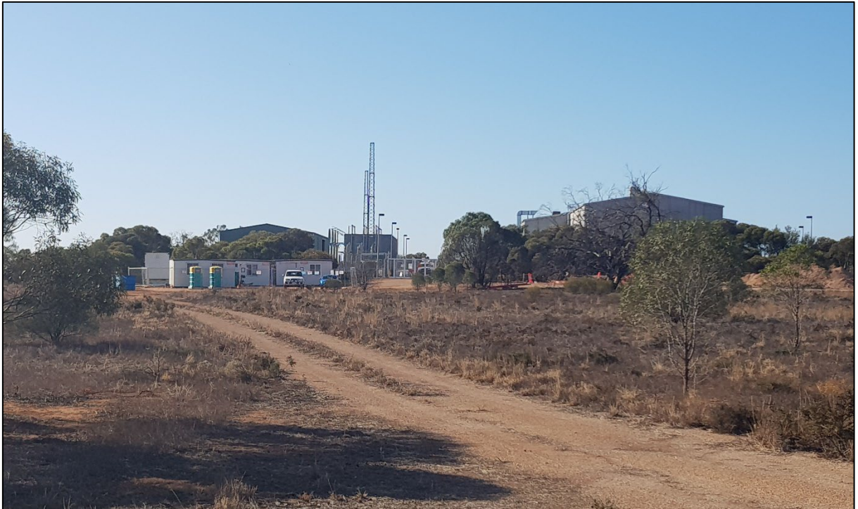
Figure 1: Murraylink Connector as viewed facing east from the Monash Substation
