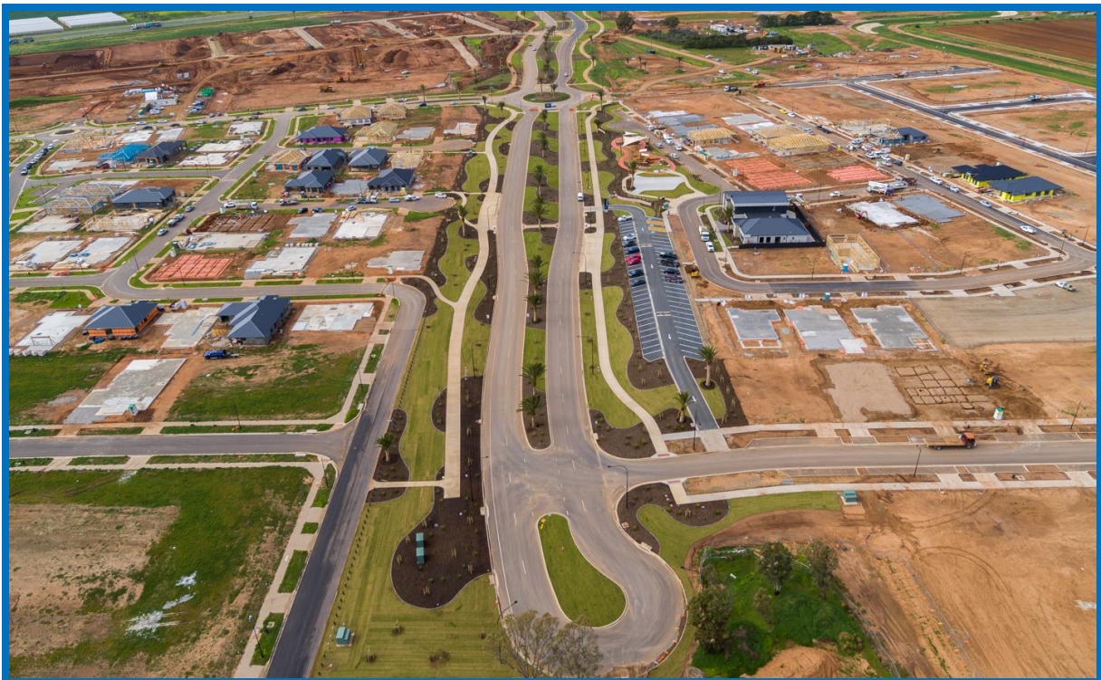
Photo 3 - Precinct 1 - Dwelling Construction (Drone Image Captured July 2022)
