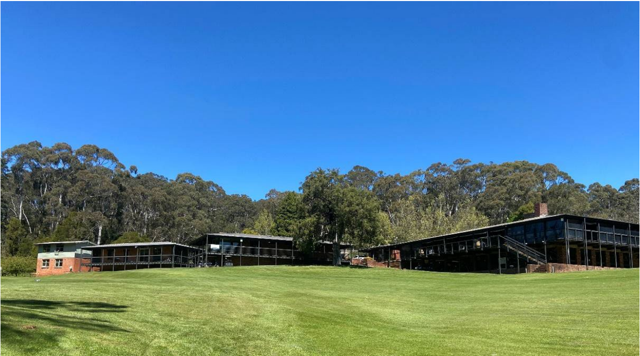
Image 2 – Existing Clubhouse Buildings
