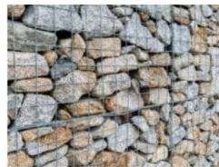
W1 - Gabion Wall - Local Stone
