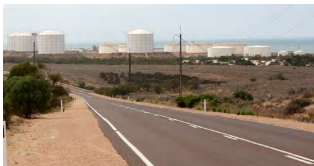
Figure 9.4c: Existing Santos Facility
