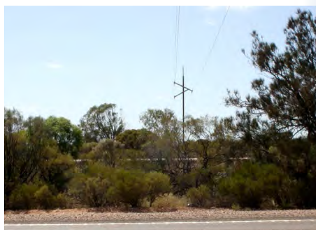
Figure 9.4b: Existing rail line running parallel to the Lincoln Highway on a small embankment
