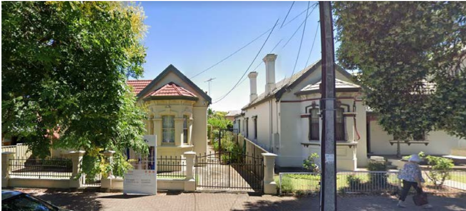
73 & 75 William Street (outside the protected historic zone). Demolished in favour of modern facilities and double garaging.
