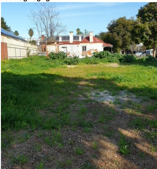
Junction Elizabeth & William St. Rear heritage building still standing, but seemingly left to 'rot'.
