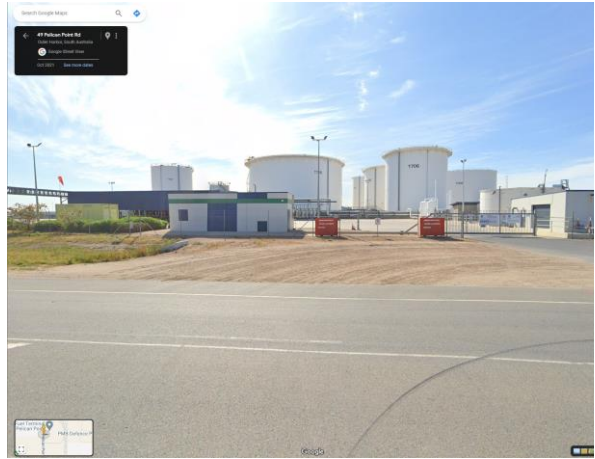
Figure 10.2.2 Ampol fuel terminal
