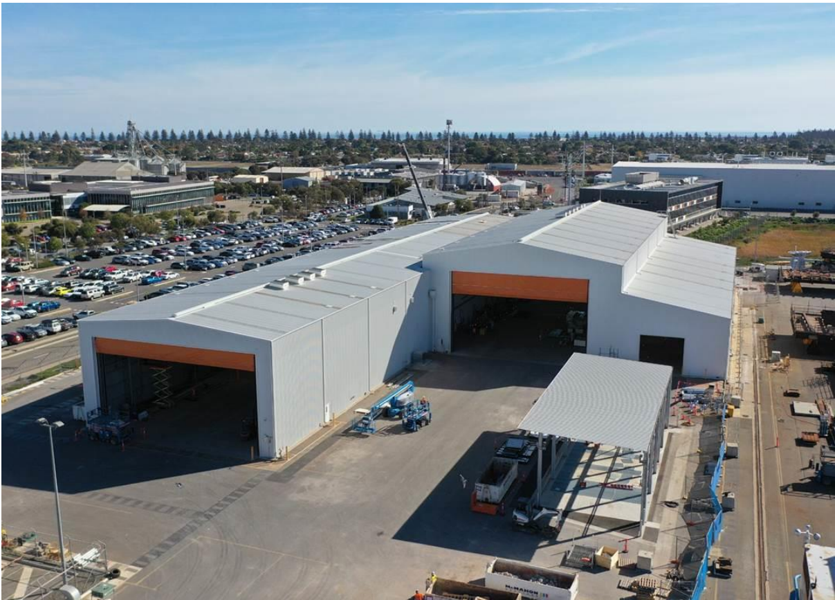
Figure 2.11 –Example of existing ONS building for manufacturing
