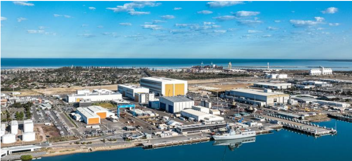
Figure 10.3 Aerial view of the existing Osborne Naval Shipyard
