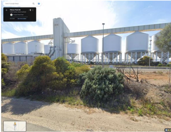
Figure 10.2.1 Viterra grain silos
