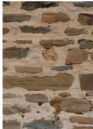
Ironstone, earthy tones with a richness and unexpected lustre. Laid with man made precision and regularity, paired with natural imperfection and irregularity
