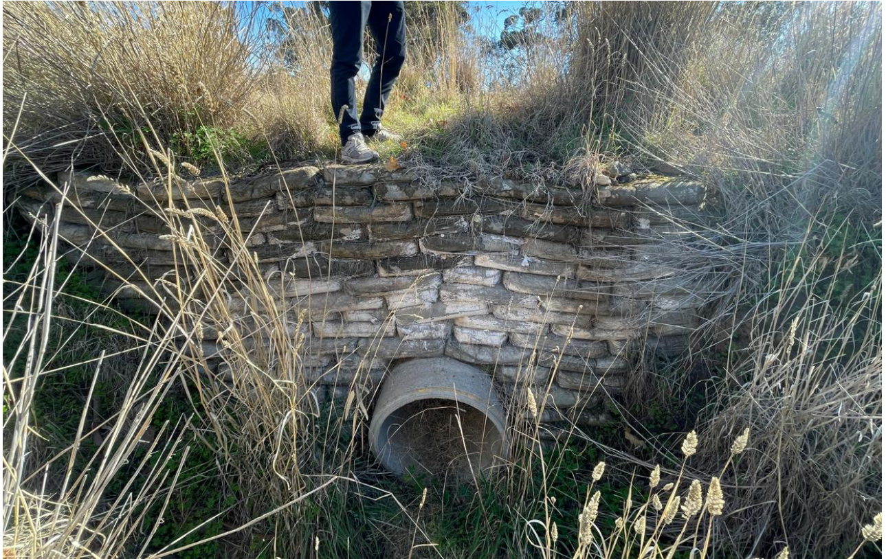
Figure 5 - Hoffnungsthal Road culvert inlet
