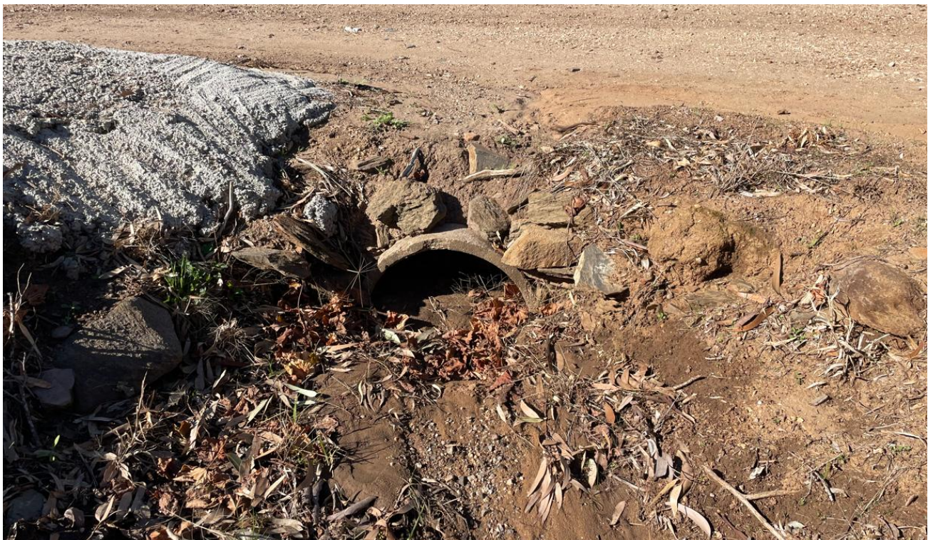
Figure 6 - Hoffnungsthal Road culvert outlet
