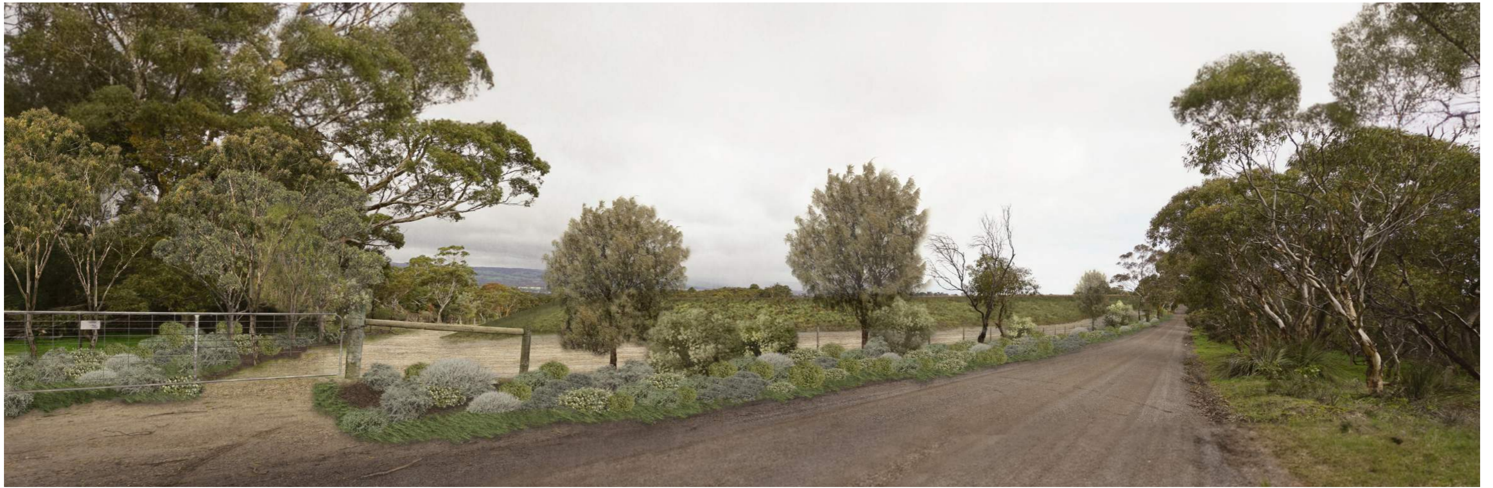
VIEW OF DAM PROJECT 5 YEARS AFTER CONSTRUCTION
