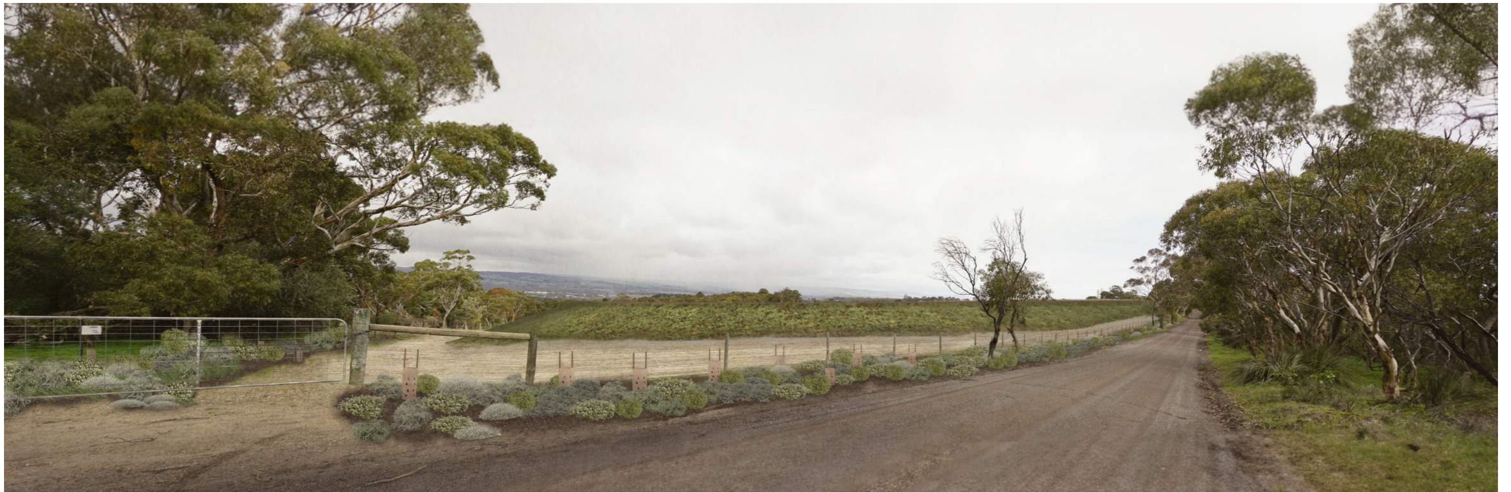
VIEW OF DAM PROJECT POST CONSTRUCTION (1 YEAR)
