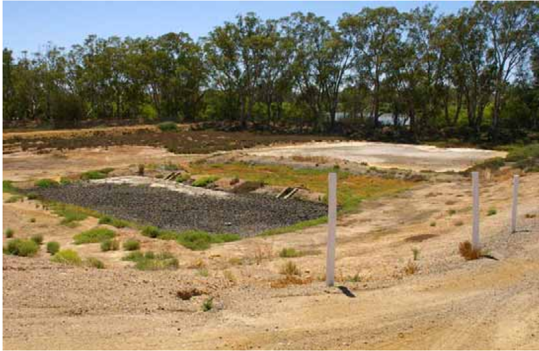
Photo 6.8 – The existing sludge drying beds
