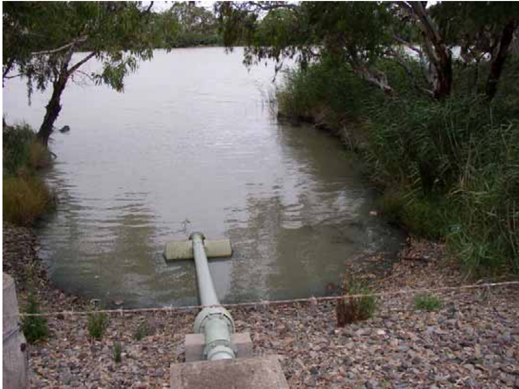
Photo 6.10 – The existing pumping suction pipe
