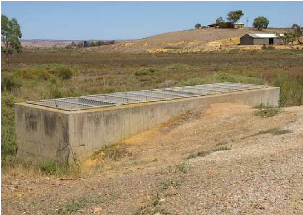
Photo 6.7 – The existing wastewater lagoons overflow structure
