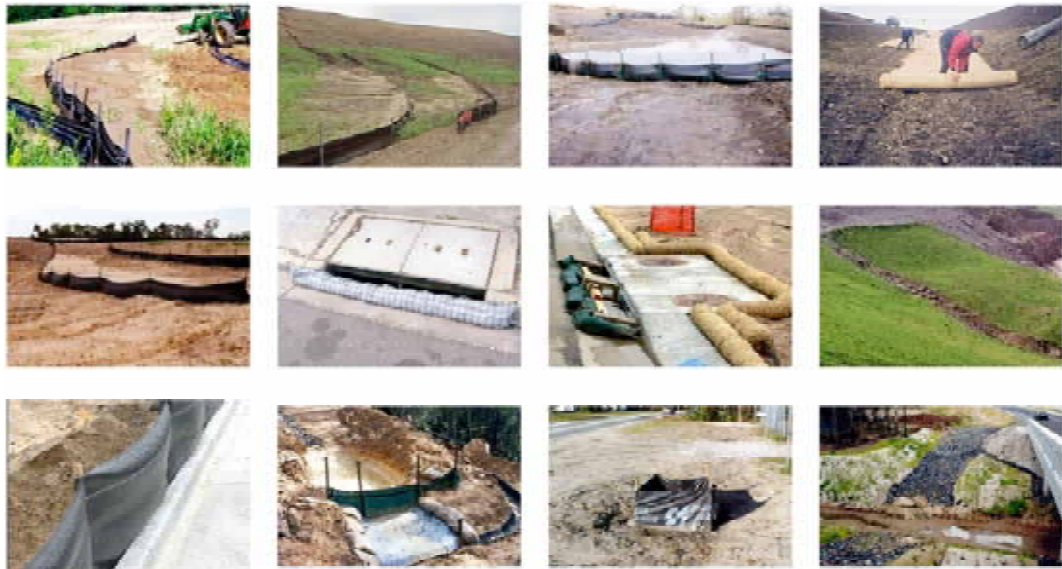
Figure 12.1 – Collage of sedimentation retention techniques
