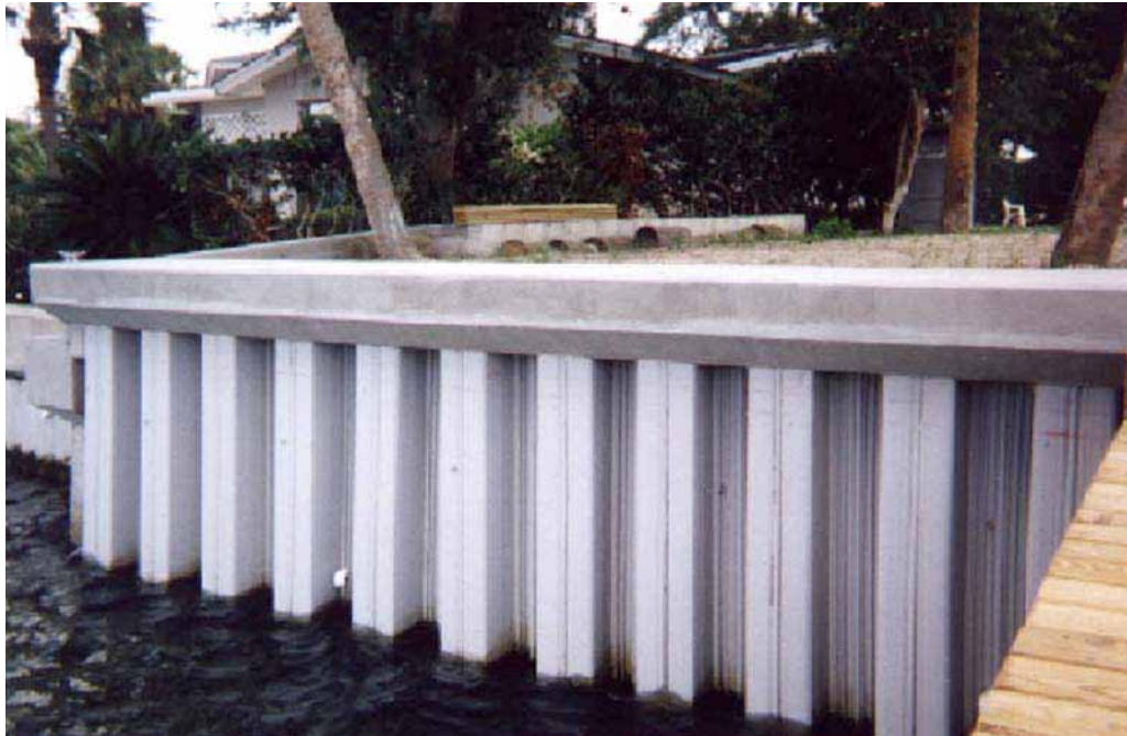
Photo 2.11 – Typical vinyl sheet piling with concrete capping
