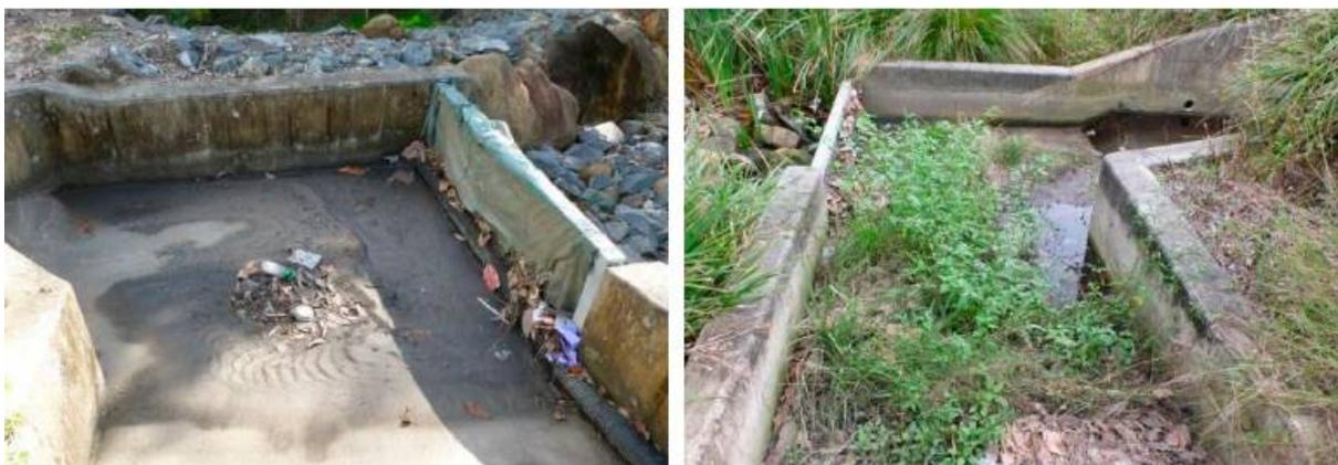
**Figure 38: Example of concrete forebays** (Appendix C3 Figure 5.4)
