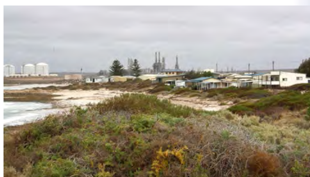
Figure 10.4d: Point Lowly coastal homes with the Santos processing facility in the background
