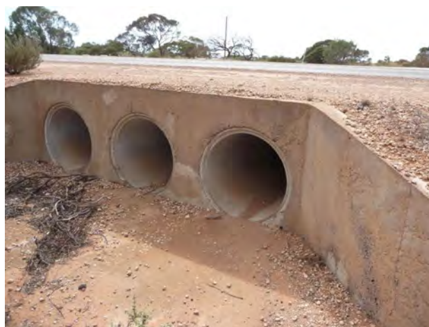
Figure 4: Culvert at turnoff to Port Bonython Road
