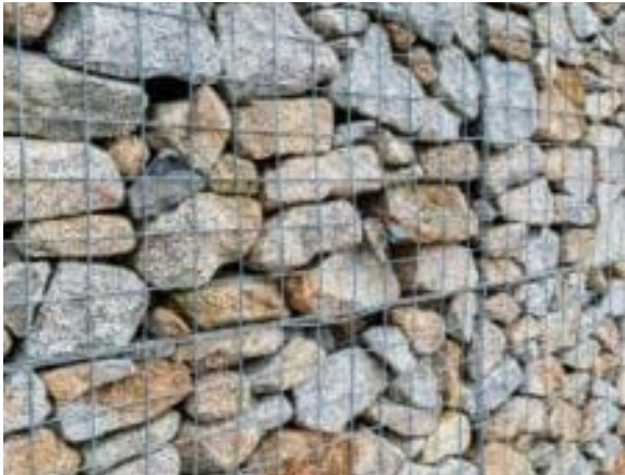
W1 - Gabion Wall - Local Stone
