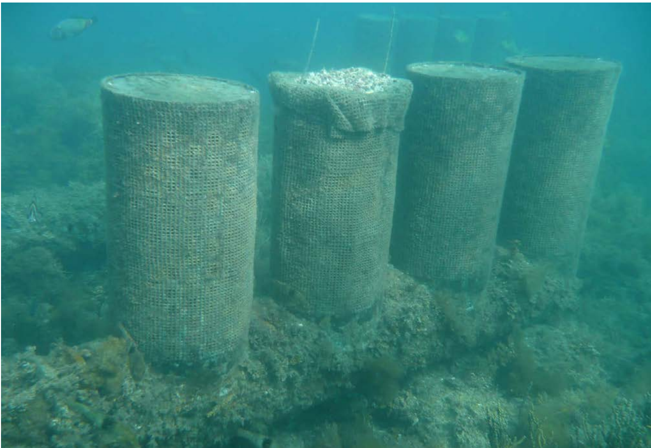
PLATE 11-1 YUMBAH SEAWATER INTAKES (RISERS) IN SMITH BAY
