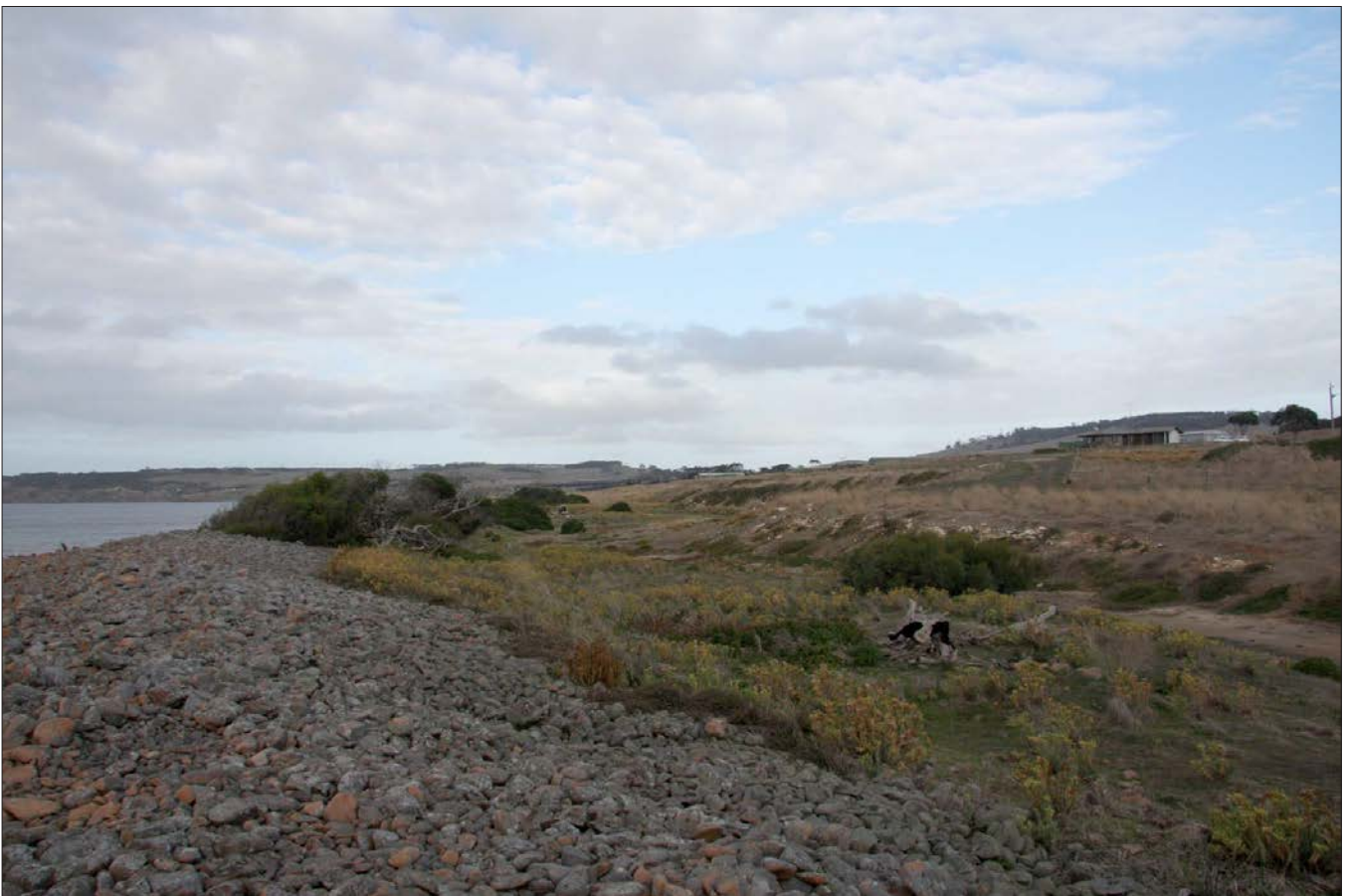
PLATE 16-3 PHOTOGRAPH ILLUSTRATING SITE SLOPE
