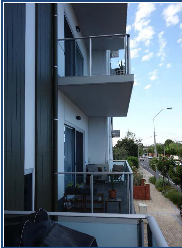
Figure 10: Lack of privacy between balconies and balconies from street level (Churchill Road, Prospect)
