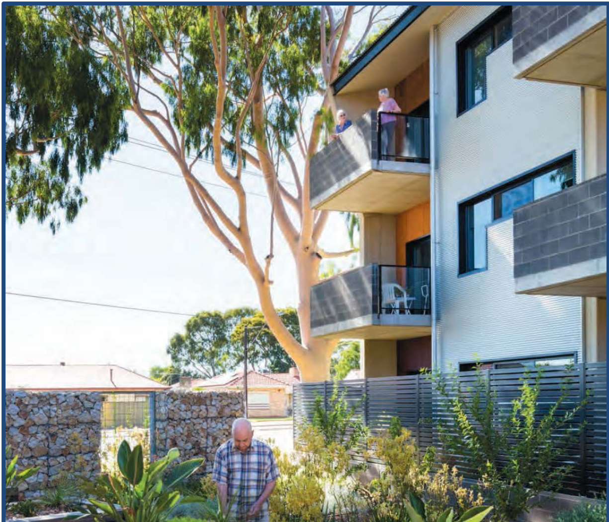
Figure 11: Well sized and functional balconies (Lumina Apartments, Somerton Park)
