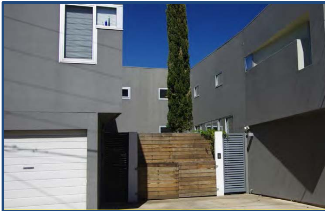
Figure 22: Screened bin store located in courtyard entry (Bowden development)
