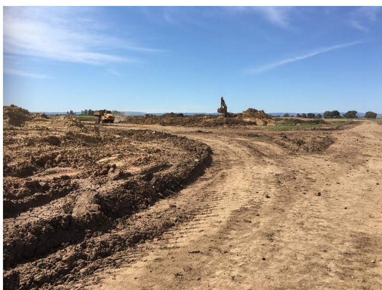
Photograph 10. Excavation of topsoil from south-eastern portion of site. 17.10.2022.
