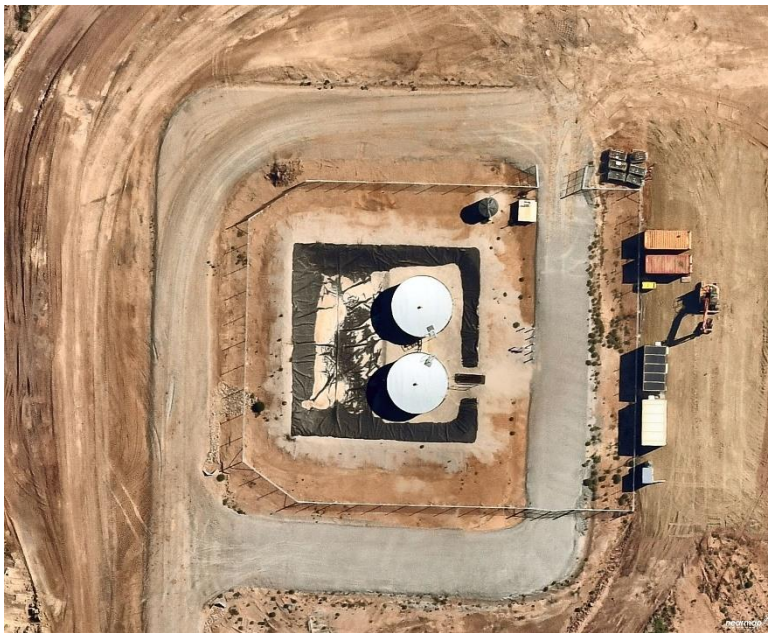
Photograph 15. Aerial view of two bunded ASTs used for temporary storage of sewage, located to the east of the site. Source: Nearmaps 09.03.2022.
