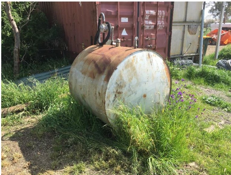
Photograph 6. Fuel AST adjacent shed at the northern site boundary. 17.10.2022.
