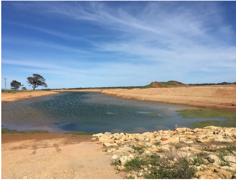
Photograph 11. View to the west of stormwater detention channel at southern site boundary. 17.10.2022.
