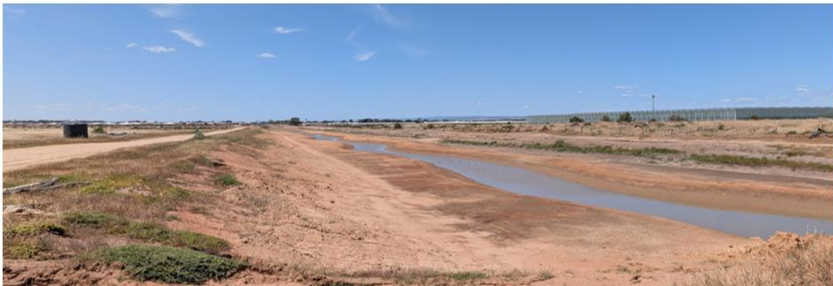
Figures 5-8 (from top to bottom), views to the north of Precinct 3A, to the north-east across Precinct 3A and to south-east across Precinct 3A. The final photo being the existing stormwater drainage channel/basin, parallel to Legoe Road, which will eventually discharge to Thompson's Creek.
