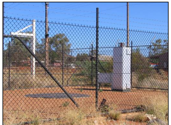
Stand Pipe & Sewer Pump Station
