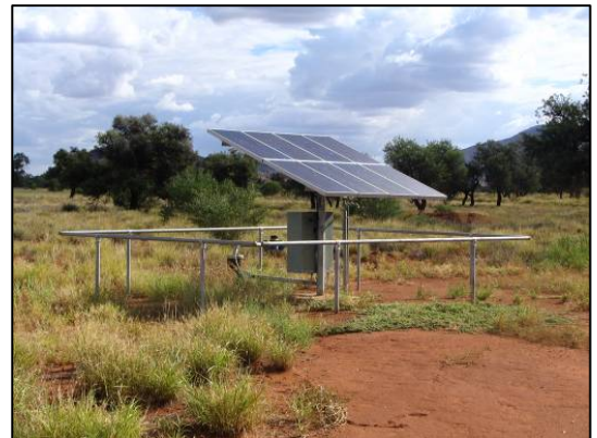
Water Bore (Solar)
