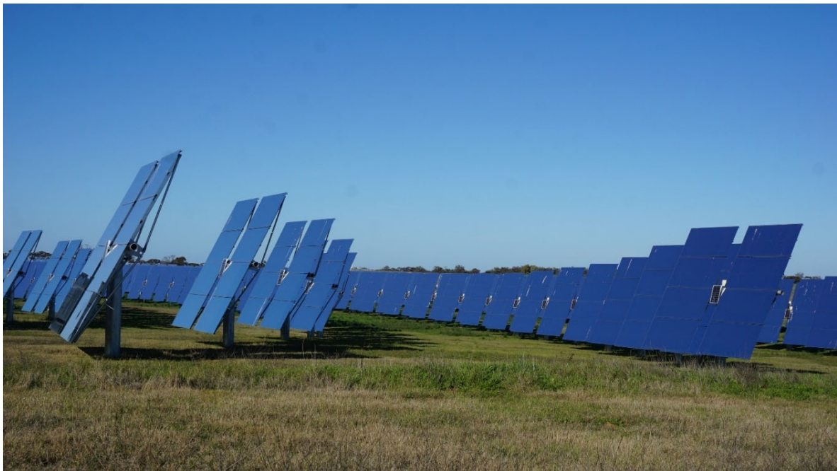
Figure 15: Heliostat in operation with mirrors facing the receiver at RayGen's Carwarp demonstration facility.
