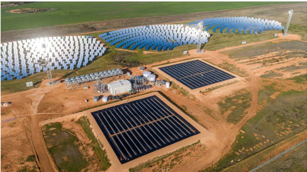
Figure 11: RayGen commercial demonstration facility Carwarp, Victoria – Source photograph RayGen
