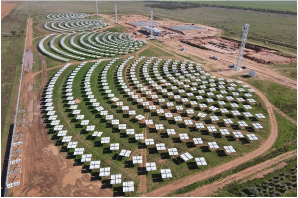
Figure 6: RayGen commercial demonstration facility Carwarp, Victoria – Source photograph RayGen
