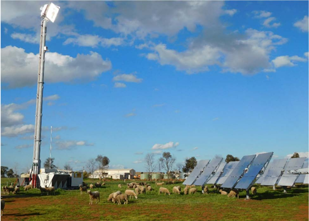
Figure 29: Sheep grazing at RayGen's renewable energy facility at Newbridge, Victoria.
