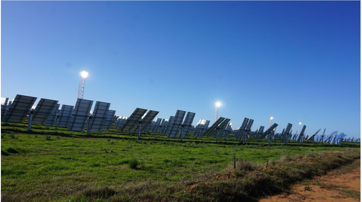
Figure 19: Halo effect of receivers at RayGen's demonstration facility at Carwarp Victoria.
