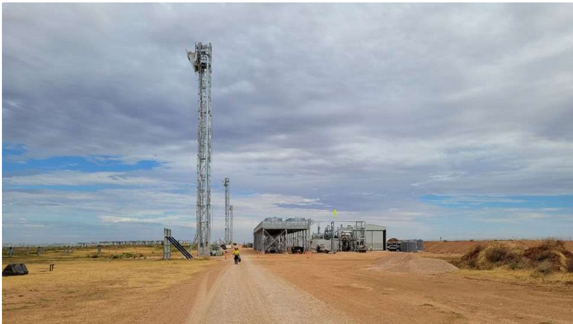
Figure 3: View of heliostats, receivers and hydro thermal plant and equipment at RayGen site, Carwarp, Victoria.
