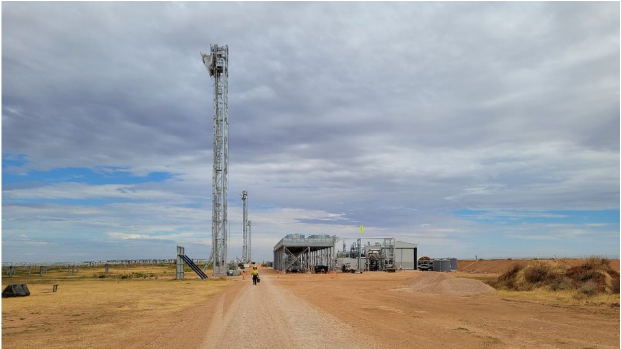
Figure 10: View of heliostats, receivers and hydro thermal plant and equipment at RayGen site, Carwarp, Victoria.
