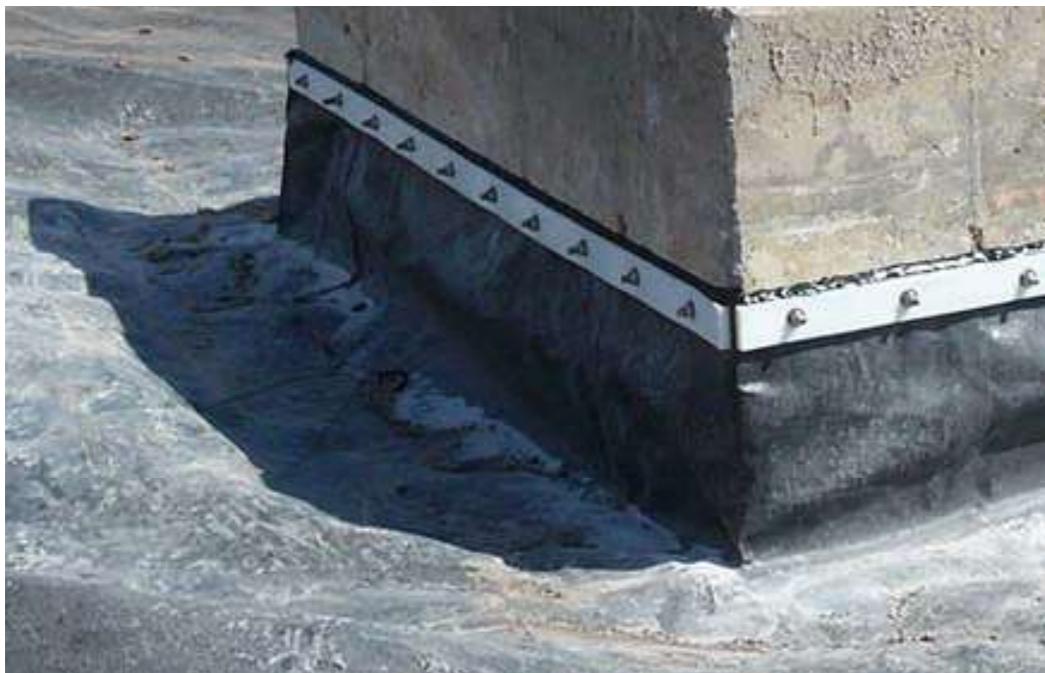
Indicative Polylock/termination bar fixing
