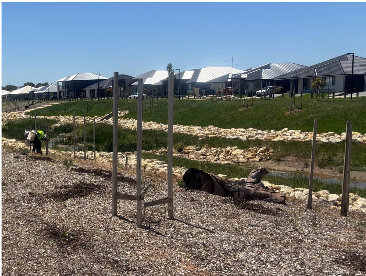
Photo 1 –Landscaping works in Stormwater Channels (including the use of felled trees)
