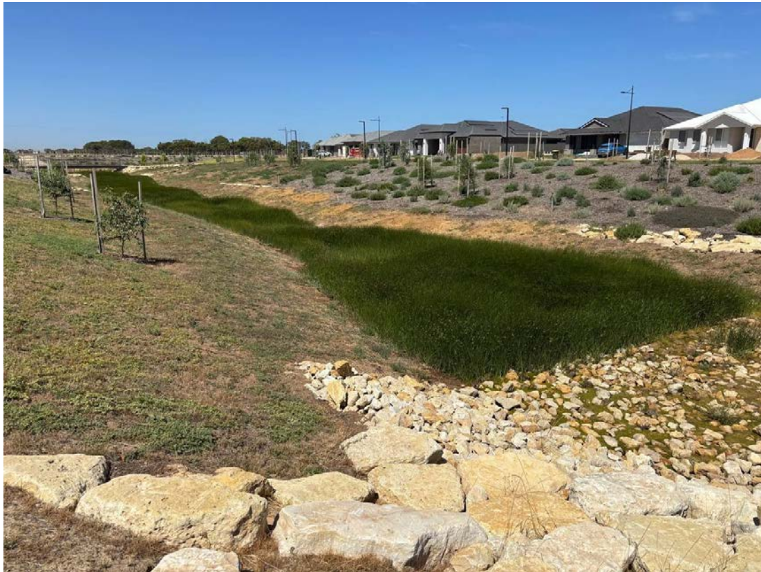
Photo 2 –Landscaping works in Stormwater Channels
