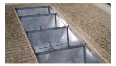
Figure 5-1: Example of Burnley Baffle technology used for dust mitigation at truck unloading bays
