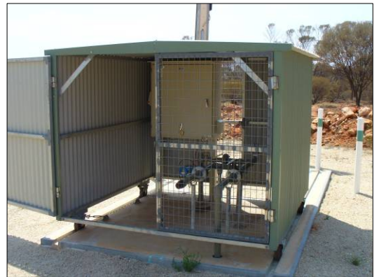
Water bore pumping equipment
