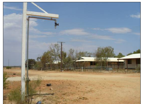
Water tanker filling point
