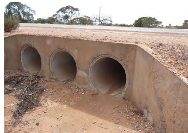
Figure 4.4c: Culvert at turnoff to Port Bonython Road
